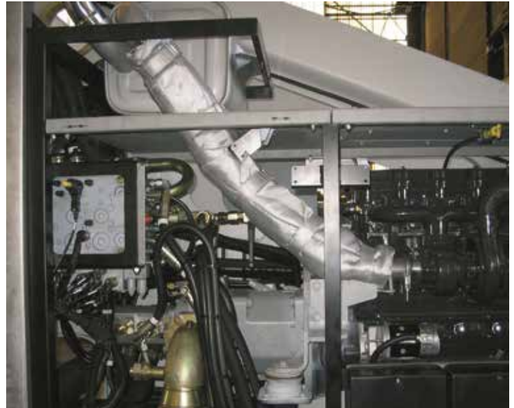
Exhaust gas insulation
