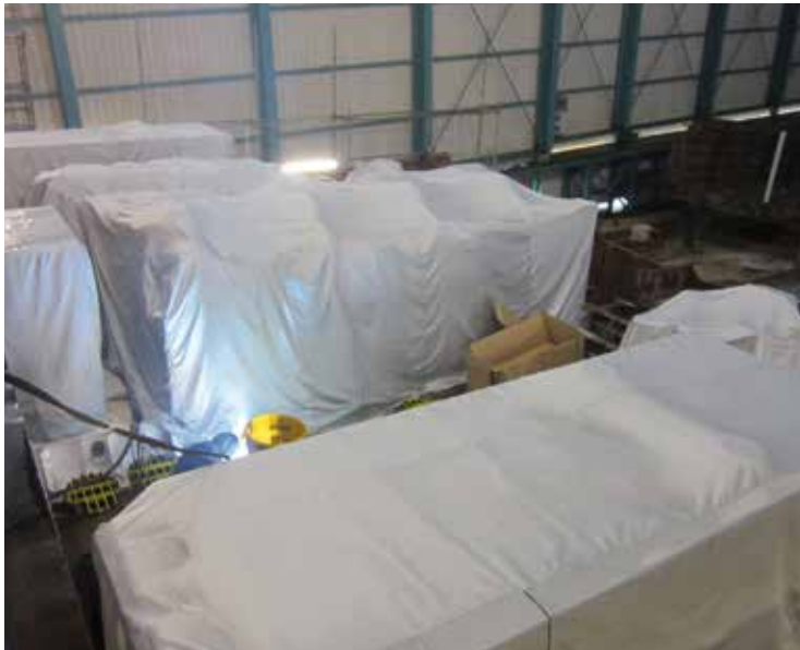
Equipment jacking in shipyards during welding work
